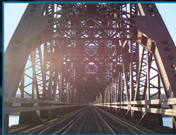
Bridge Timbers & Panelized Decks
